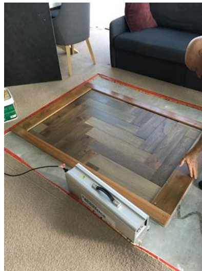
Figure 1: Testing in the living room of Unit 1501
